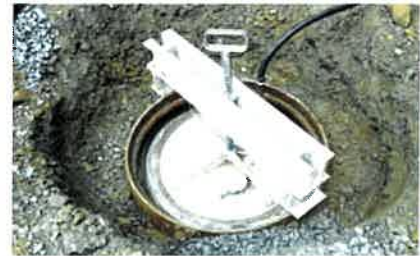
New SMH vacuum testing
