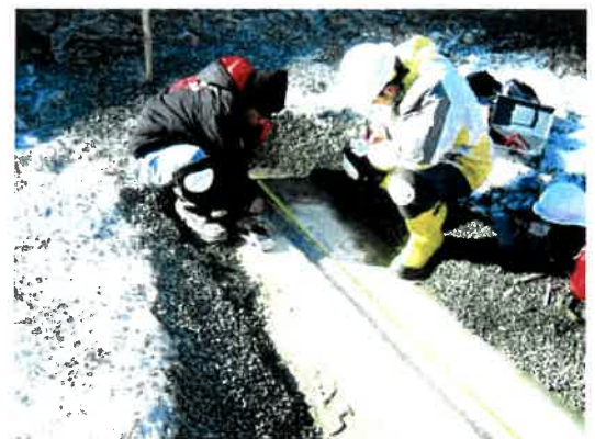
Exterior resistivity testing
